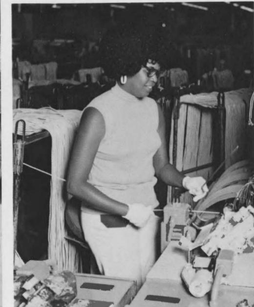
*Top Right:* Telephone cords, used to connect telephones to baseboard outlets, are manufactured in Baltimore and Buffalo.
