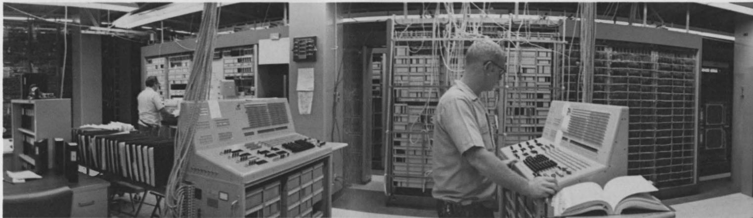
*Top Left:* WE personnel install the first of a new frame system called Cosmic-Cosmos at the Beverly Hills, Calif., central office. The new system helps maintain order in the maze of wires coming into a central office and helps the telephone companies realize savings in both wiring and clerical costs.
