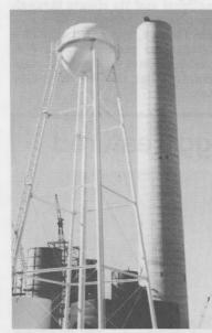
CHIMNEY TOPPED: Pullman Kellogg's chimney group recently topped out this 385-foot-tall jump-formed concrete chimney at Cochise, Arizona, and currently is installing two steel liners inside the chimney. To erect the structure, the utility's water tower had to be moved in one piece a distance of approximately 500 yards.
