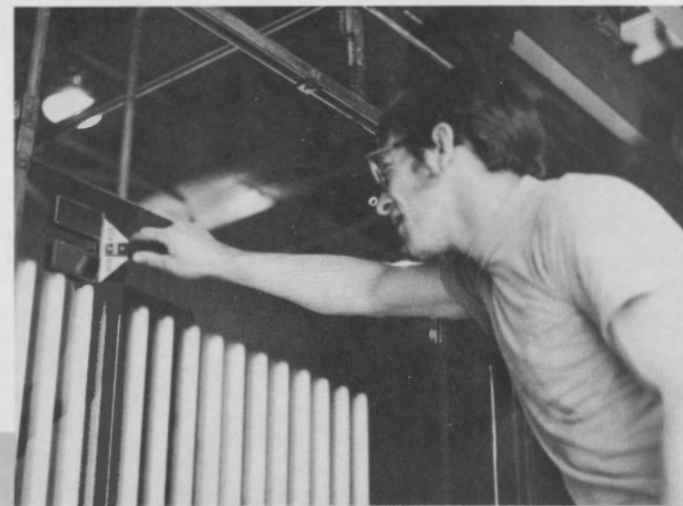
The color of each Vari-Tran reflective glass panel must meet exacting specifications. Dave Ruffert uses a paddle and background lights to check the color of a newly coated panel. The paddle holds two Vari-Tran samples—one with the coating too dark, the other too light—and the panel's color must be exactly between the two.
