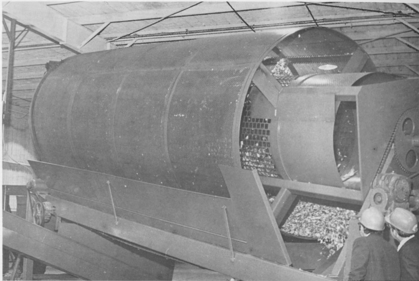
This end view of the drum screen shows processed chips being run to the conveyor while finer screened chips are conveyed to the opposite end of the drum for further processing through the rotary screen.
