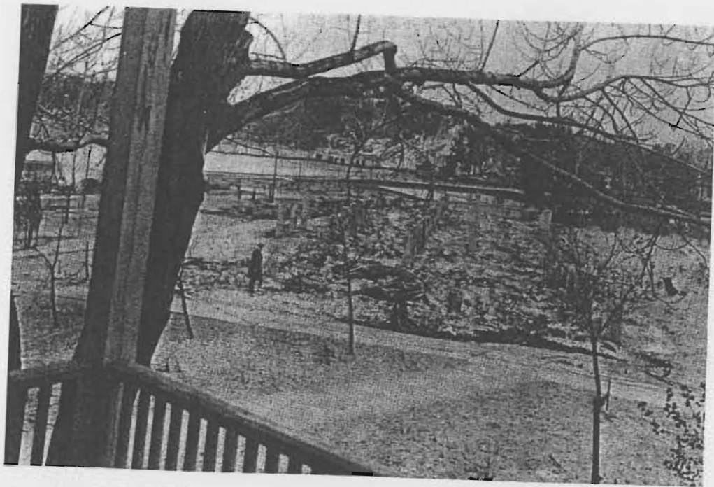
The ruins of the Ottawa Beach Hotel Annex as seen from the veranda of the Pantlind Cottage. Some of the concrete pilings were still on the hillside in 1986.
