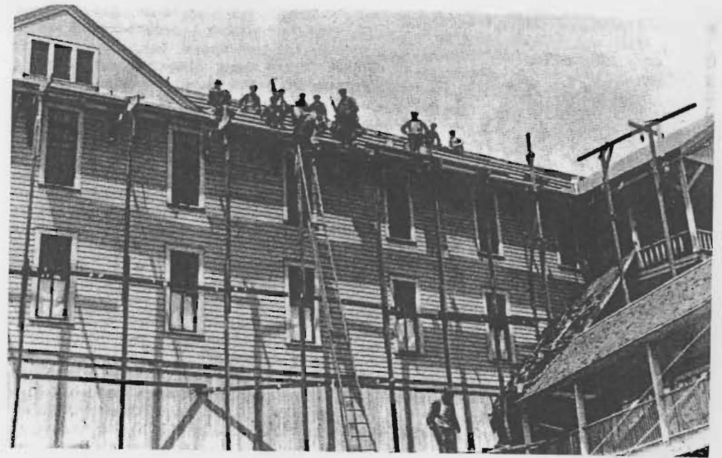
Reroofing the Annex in the summer of 1923. The Annex was also painted.
