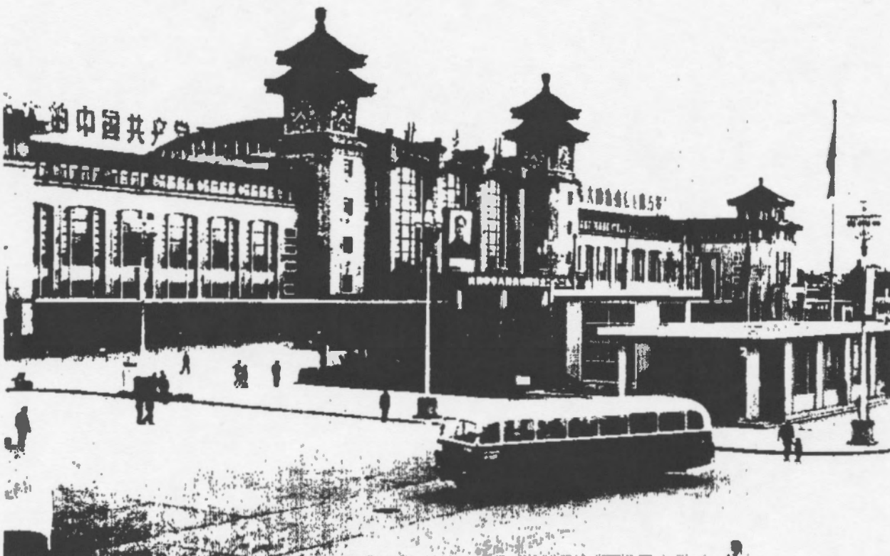
Figure 31. The Peking Railroad Station. The subway now traverses the area beneath the square in front of the station.
