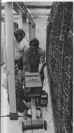
Top Left: WE personnel install the first of a new frame system called Cosmic-Cosmos at the Beverly Hills, Calif., central office. The new system helps maintain order in the maze of wires coming into a central office and helps the telephone companies realize savings in both wiring and clerical costs.
