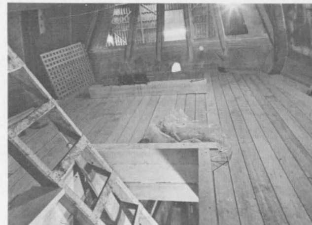
August 1976: The main deck extends aft into the great cabin, where a hatchway leads to the engine compartment below.
