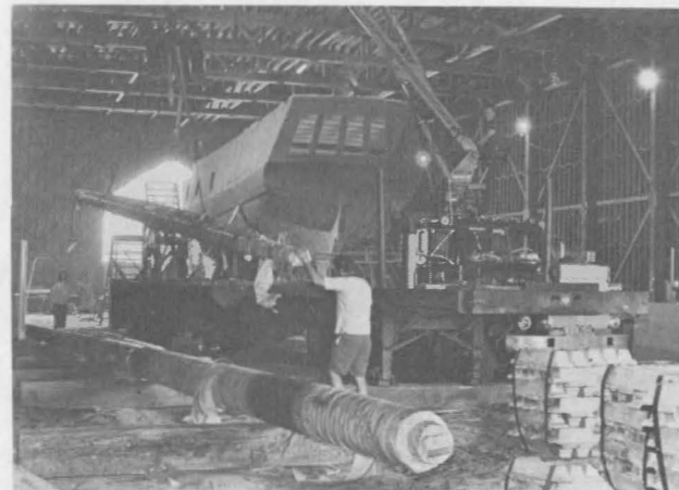
Huge timbers of Douglas Fir for mast, boom and other spars are shipped in from Oregon.
