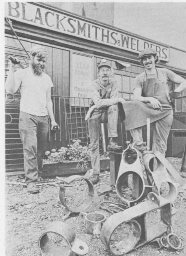
August 1976: Heavy metal fittings for the spars and the hull are fashioned by skilled craftsmen working in the traditional manner in a blacksmith's shop on Newport's waterfront.
