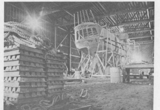
September 1976: Nearing completion, the vessel is being prepared for painting and installation of rudder and propeller. Lead ballast (total 33 tons) and cordage (left foreground) await placement.
