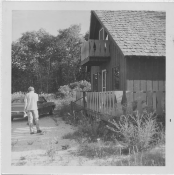
Fig. 5 - Abandoned gift shop owned by Mrs. Bloomer on west side of Lake Shore Drive about \frac{1}{2} -mile north of Ludington Project. Owner claimed building foundation shifted by vibration from pumping operation of turbines or underseepage.
