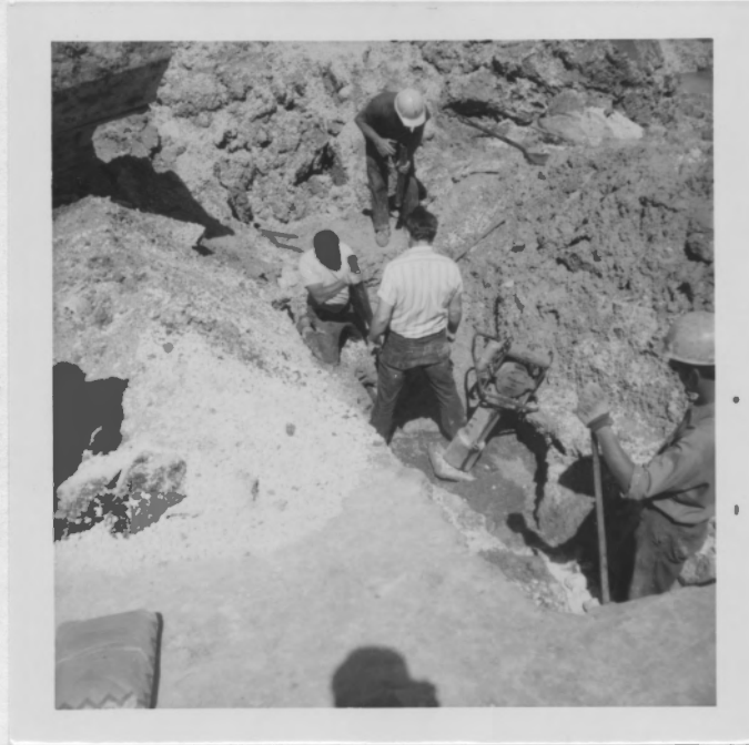
Fig. 27 - Workmen compacting backfill material in trenched-out area of lining failure (sta. 268 + 45).
