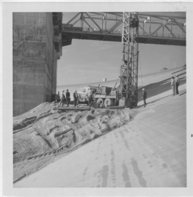
Fig. 24 - Close-up view of drilling in operation.
