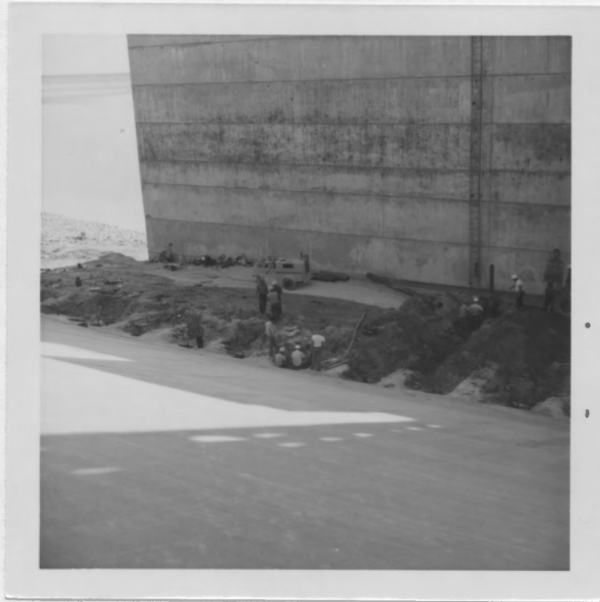
Fig. 25 - General view of well point placements taken from top of intake structure.
