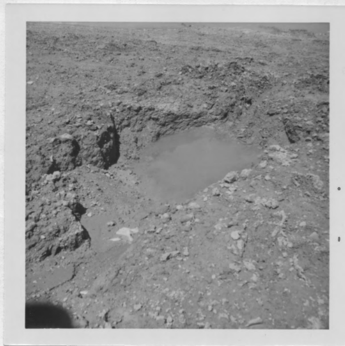
Fig. 31 - General view showing location of sink hole and area of lining failure. Photo taken from embankment crest.
