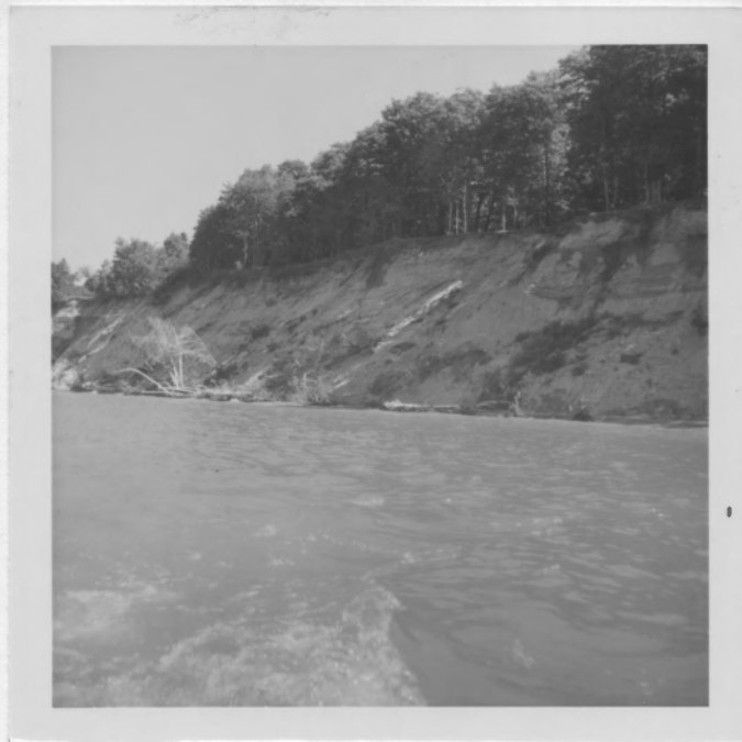
Fig. 12 - Typical slope about 2½ miles north of Ludington Project.
