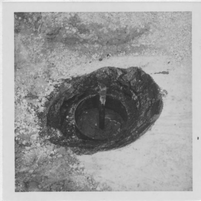
Fig. 26 - Close-up view of 18-inch casing at surface level of well point. Hot mastic material used to cap and seal opening.
