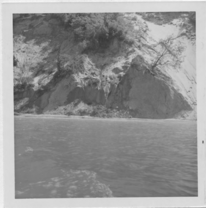
Fig. 14 - Photo depicts instability of slope. About 2 miles north of Project. Fallen trees on narrow beach at lake level.
