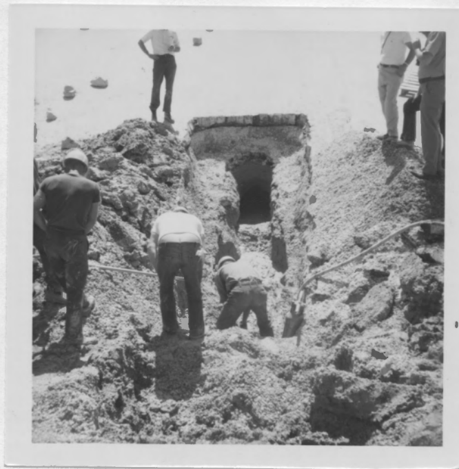
Fig. 28 - Same as Figure 27, but looking upward toward embankment slope.
