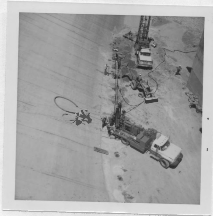
Fig. 21 - Rig drilling holes for installation of well points.
