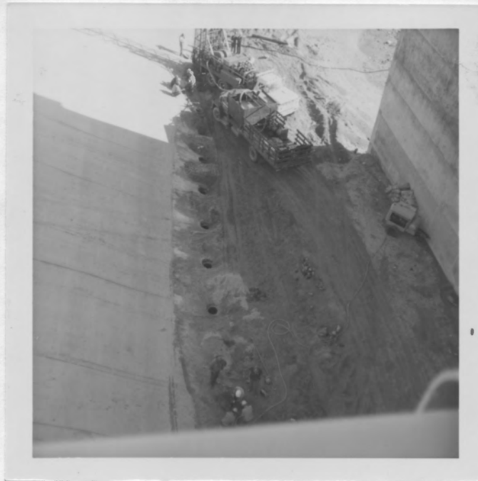
Fig. 21 - Rig drilling holes for installation of well points.
