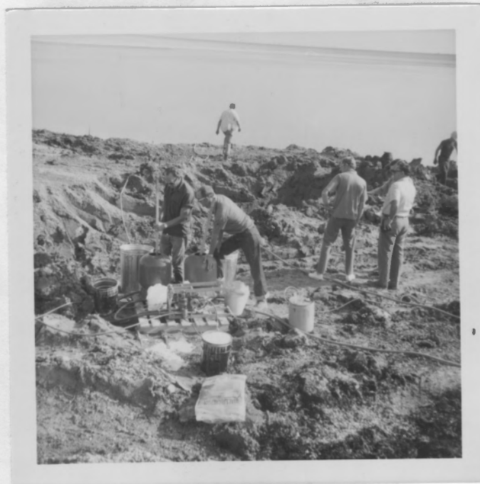
Fig. 30 - Mixing of chemical grout to fill void.
